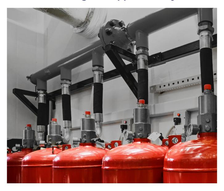
LIFECO 5112 is a Clean Agent Fire Suppression System with FK-5-1-12 (Dodecafluoro-2-methylpentan-3-one). FK-5-1-12 agent is another widely used extinguishing clean agent. It is environmentally safe and best used in fire hazard areas containing A, B, & C classes of fire.
